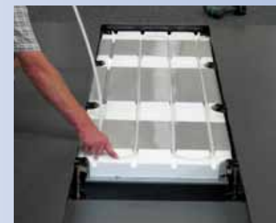
4. Installation of the heating tubes.
