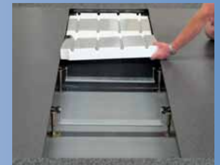
3. Installation of the heating units with heating transmission sheets.
